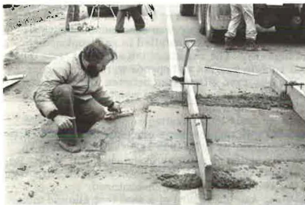
Dummy frame installed in roadway
