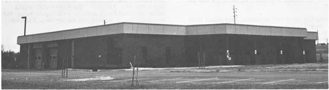
Figure 1. Exterior view of Auto Check facility, Huntsville, Alabama.
