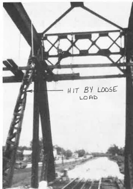
Figure 14. Notch caused by impact from loose shipment.
