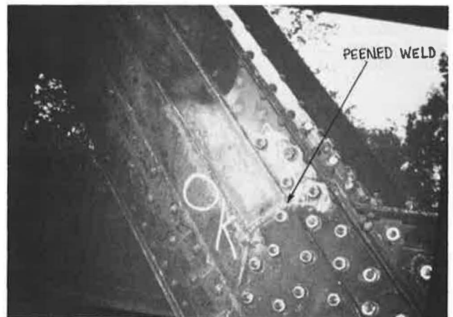
Figure 23. Truss repaired by welding and peening.
