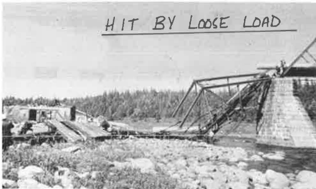
Figure 15. Truss collapse caused by impact from loose load.
