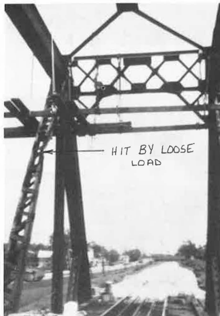
Figure 14. Notch caused by impact from loose shipment.
