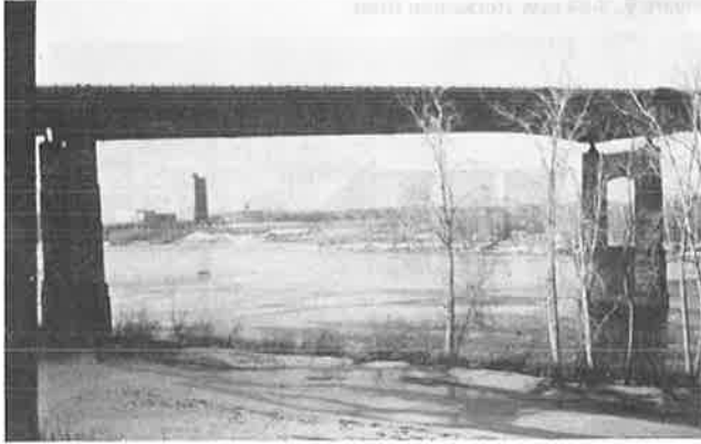
Figure 10. Charter Oak Bridge over Connecticut River.
