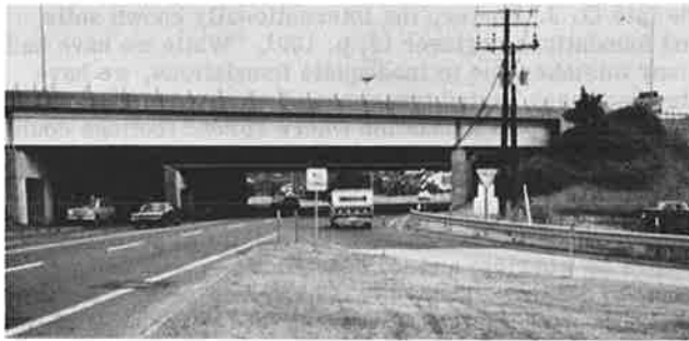
Figure 1. I-91 over Silas Deane Highway.
