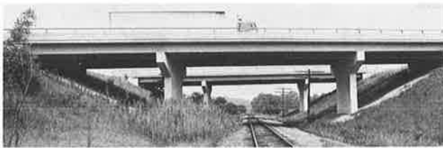
Figure 1. Steel beam bridge—continuous over piers.
