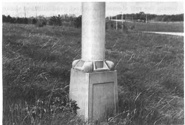
Figure 3. Typical aluminum frangible-base luminaire support.
