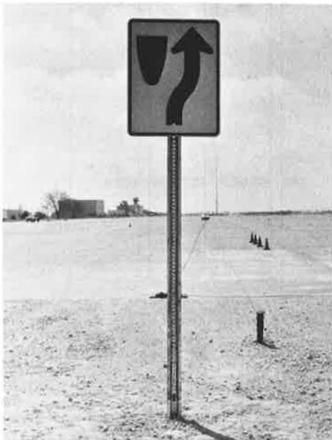
Figure 4. Single-post sign installation.
