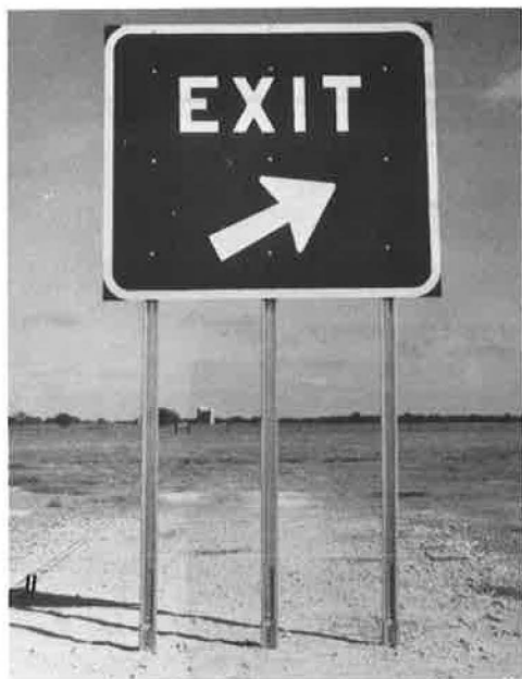
Figure 7. Three-post sign installation.
