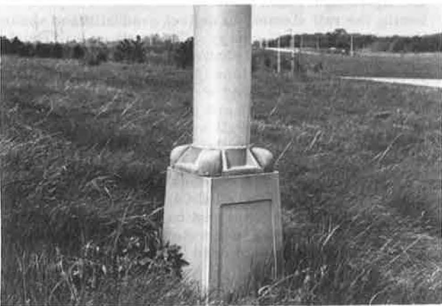
Figure 3. Typical aluminum frangible-base luminaire support.
