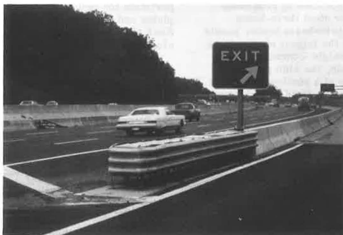
Figure 3. G-R-E-A-T system installed at end of guardrail.
