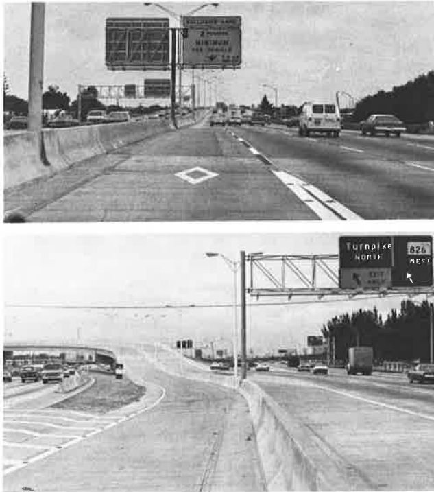
Figure 1. Views of I-95 priority-lane system.
