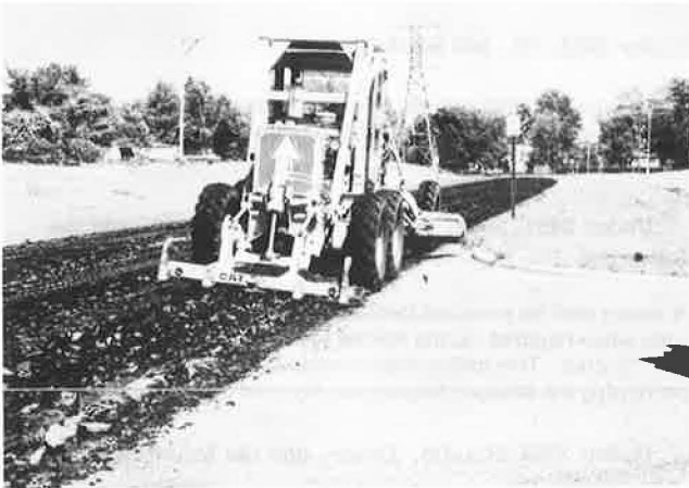
Figure 1. Motor grader ripping up old bituminous pavement for recycling.
