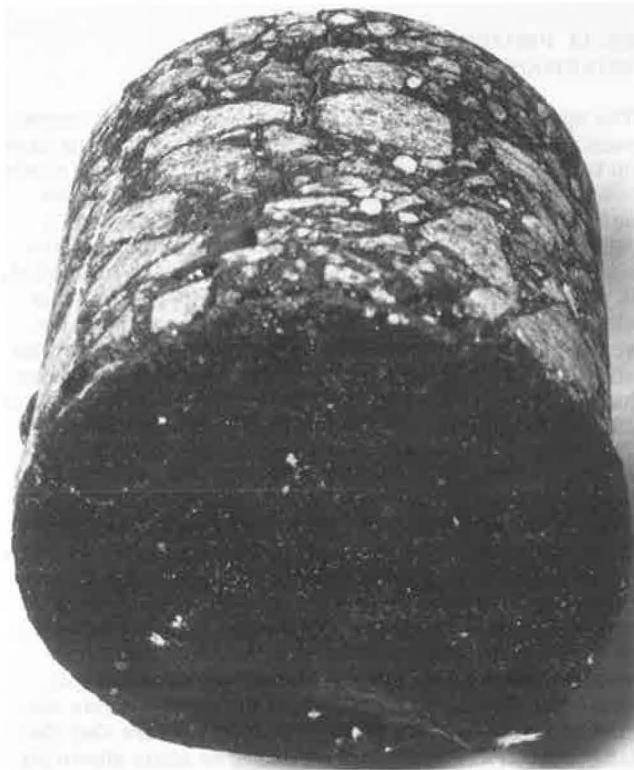
Figure 4. Core through bituminous layers and polypropylene fabric: I-95 project.
