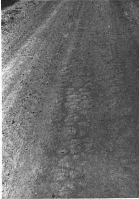
Figure 4. Stabilised Unsealed Road Surface
