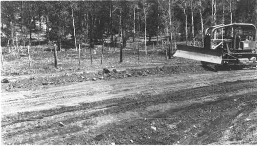
Figure 6. Windrow before and after processing by the RB-4 and the same spot about 3 weeks later. This windrow is smaller than the maximum which can be handled, but is otherwise typical. This section was not ripped.
