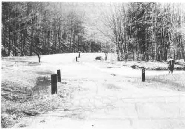
(c) Overflowing vented ford.
