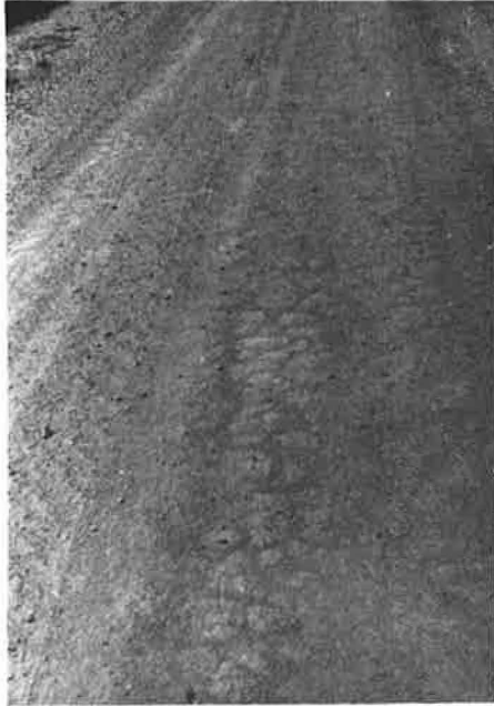
Figure 4. Stabilised Unsealed Road Surface
