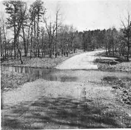
(b) Vented ford (or dip with culvert) on the White Mountain N.F., New Hampshire.
