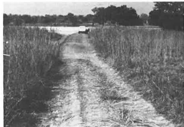
Feeder road, earth surface.
