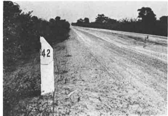
Primary road, gravel surface.
