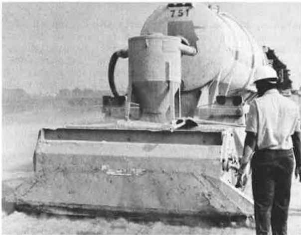
Figure 15. Spreading portland cement in regulated quantities.
