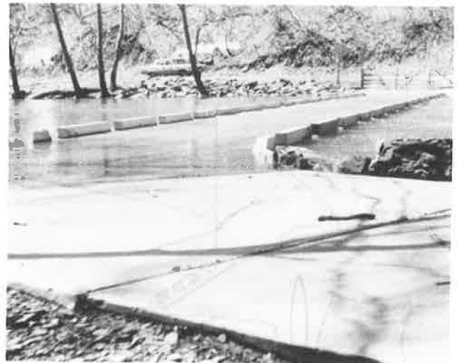
(b) Low water bridge overflowing on the Monongahela N.F., West Virginia
