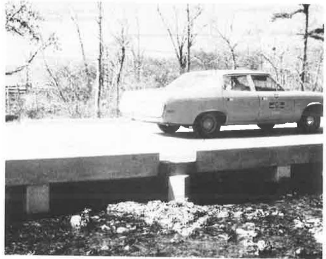
(b) Low water bridge overflowing on the Monongahela N.F., West Virginia
