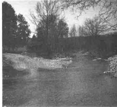
(b) Gabion ford on the Monongahela N.F., West Virginia.
