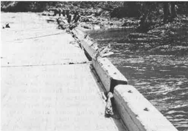
(c) Displacement caused by ice flow, water pressure and erosion.
