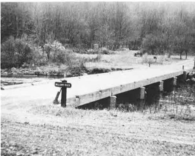
(c) Low water bridge on the Monongahela N.F., West Virginia
