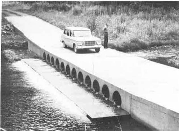
(c) Overflowing vented ford.
