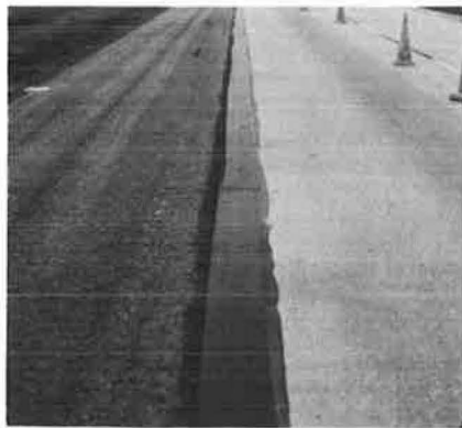
Figure 9. Sealed pavement edge joint on test section I2.
