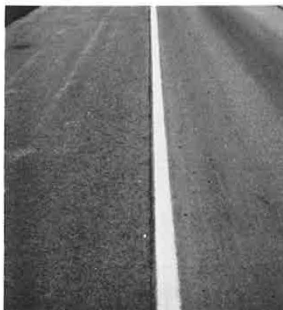
Figure 8. Pavement edge joint on test section I2.
