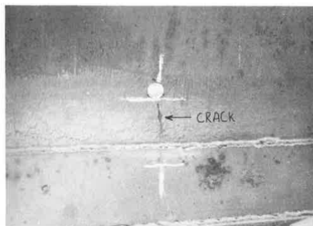
Figure 20. Inside of girder before core was drilled.
