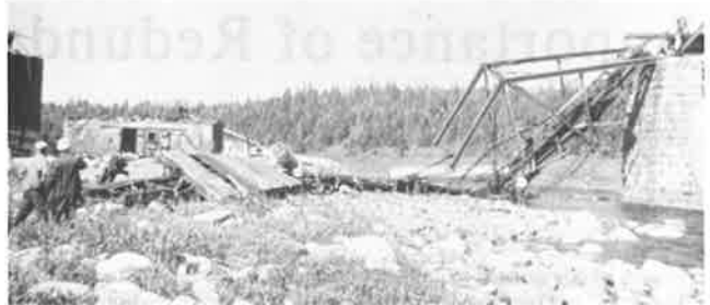
Figure 5. Result of inadequate bracing.
