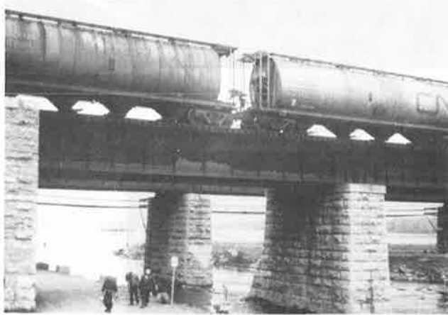
Figure 13. Girders with a Pratt truss.
