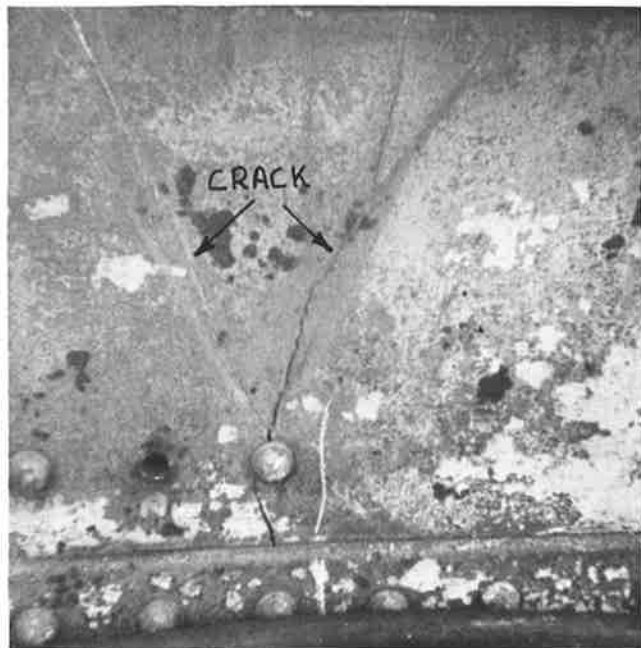
Figure 7. Crack developed three weeks after deck fire.
