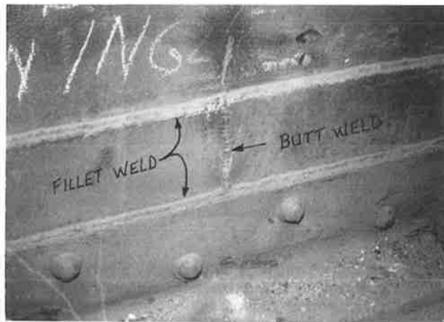
Figure 14. Butt and fillet welds.
