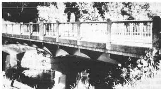
Figure 4. Ontario-35 bridge at Minden.
