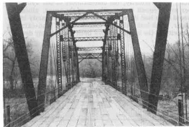
Figure 6. Hubby bridge over the Des Moines River.
