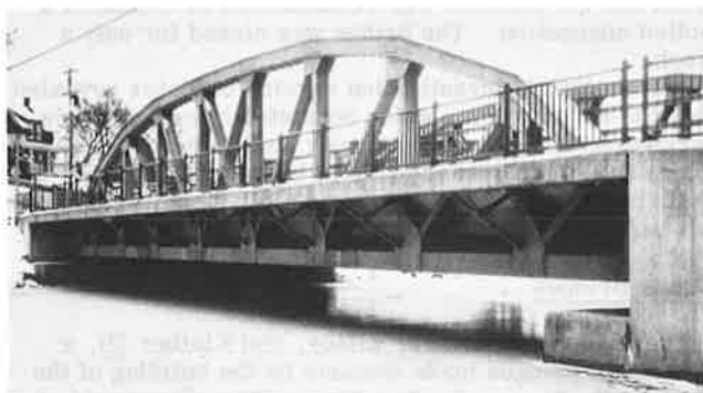
Figure 5. Ontario-33 bridge at Frankford.
