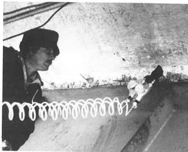
Figure 2. Epoxy injection mixed in the gun.
