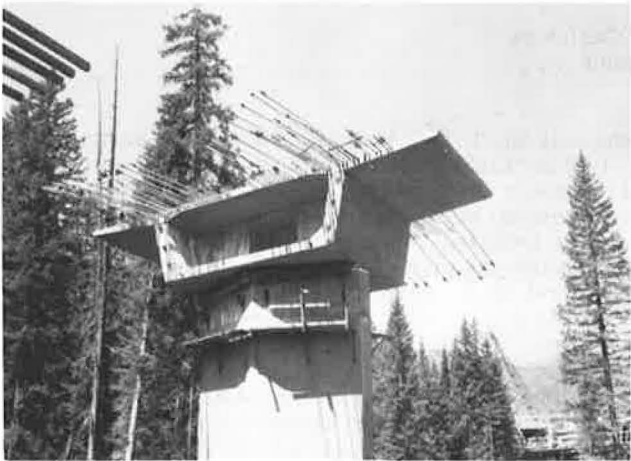
Figure 10. View of pier segment showing typical tendon arrangement: bridge AK.
