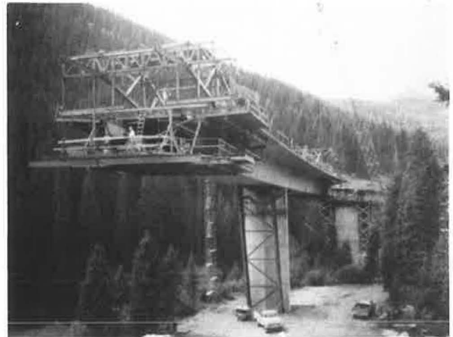
Figure 6. Free cantilevering from center pier: bridge AM.
