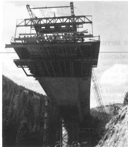
Figure 7. Bottom view of free-cantilevered span: bridge AM.
