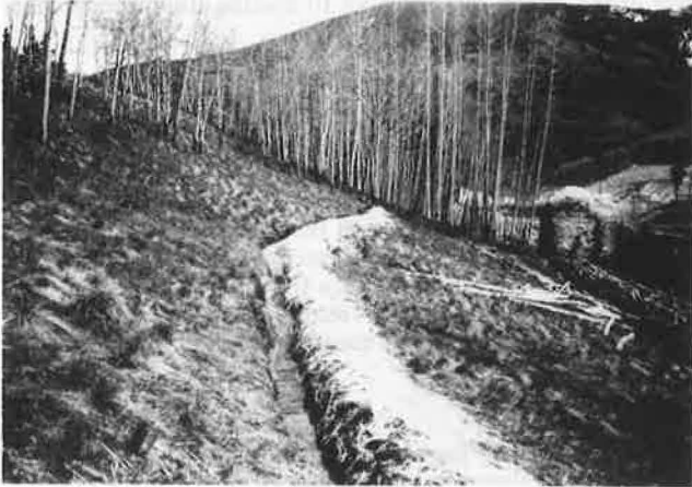
Figure 4. Hand-dug interception ditch above project area.
