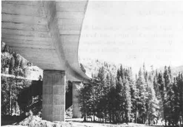
Figure 4. Precast concrete segmental box-girder bridge.
