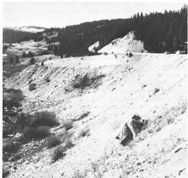
Figure 3. Old construction scar along existing highway.
