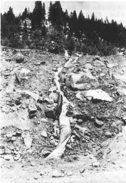
Figure 5. Failure of plastic-lined ditch.
