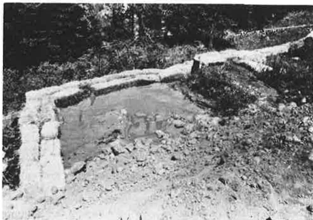
Figure 2. Straw-bale sediment trap.
