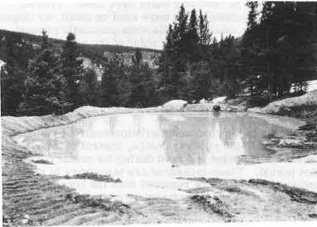
Figure 1. Excavated sediment basin.
