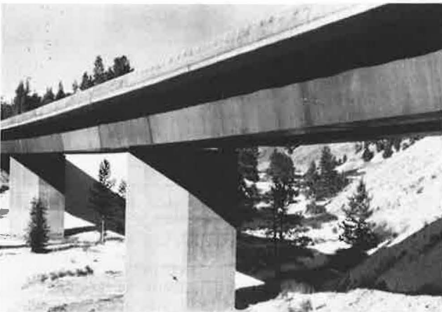
Figure 5. Typical welded box-girder bridge.
