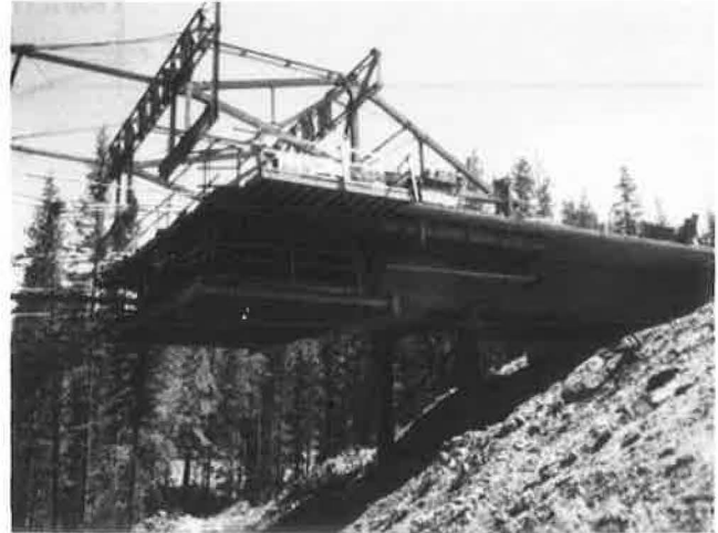
Figure 5. Side-span cantilever construction: bridge AL.
