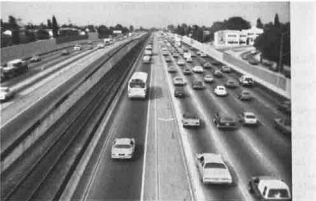
Figure 5. Eastern segment of busway.
