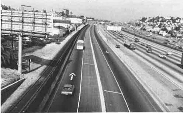
Figure 4. Western segment of busway.
