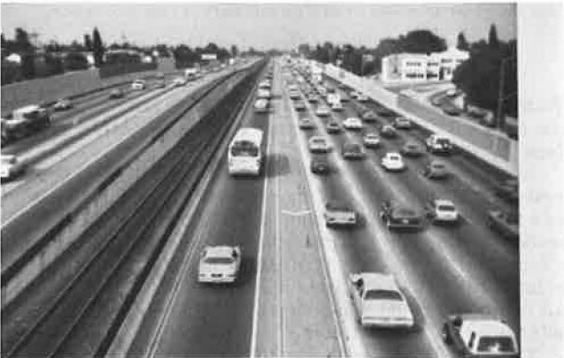
Figure 5. Eastern segment of busway.
