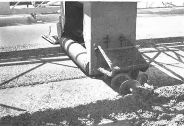
Figure 9. Poor finish resulting from a rapid loss in workability.
