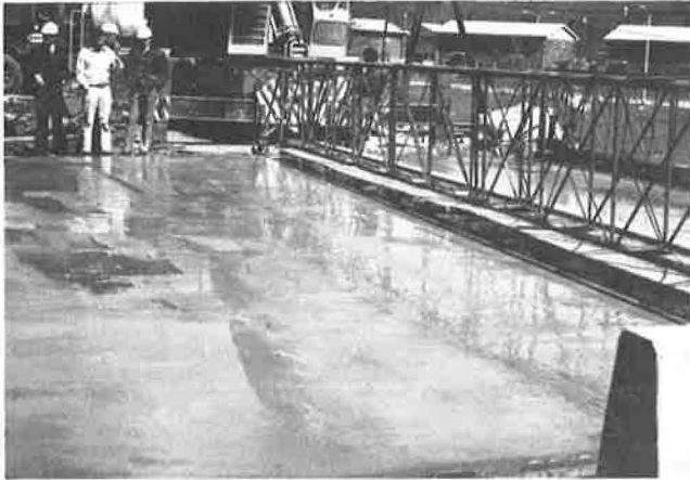
Figure 8. SWR concrete being pumped into place on I-85A.
