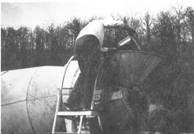
Figure 2. Liquid SWR admixture added to ready-mix truck.
