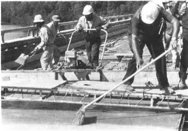
Figure 10. Satisfactory finish obtained with a vibrating straightedge and rapid placement operation.
