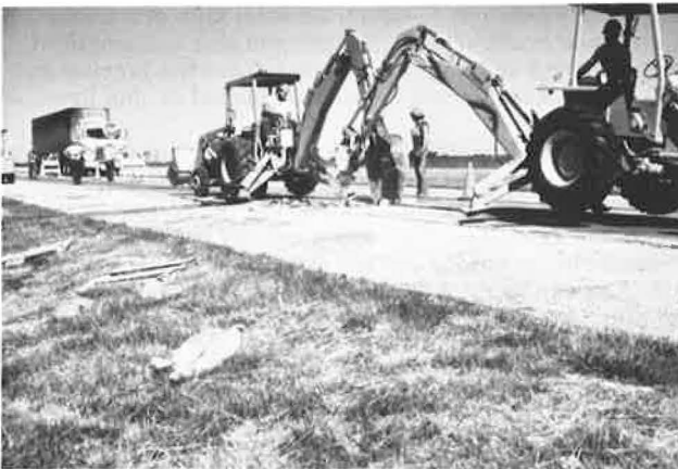
Figure 8. Hydrhammer breakout and mechanized pavement removal operation.
