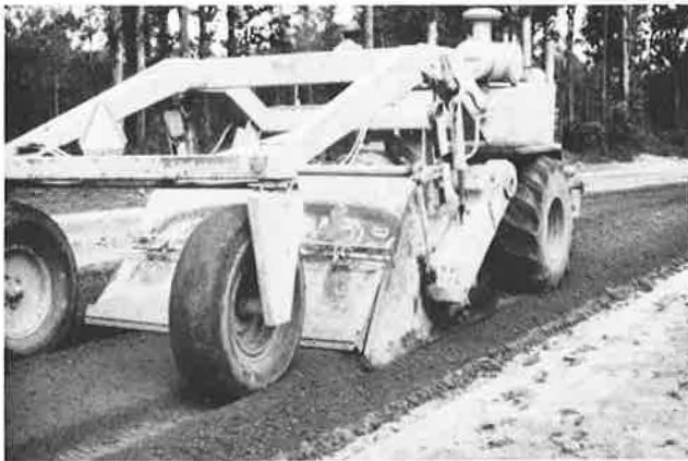
Figure 2. Soil-cement mixing on Louisiana project.
