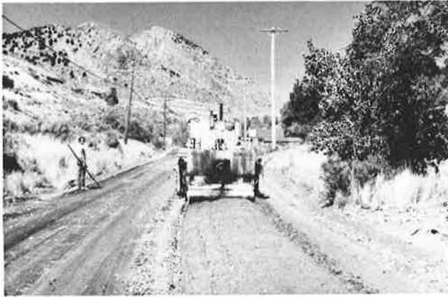
Figure 1. Breaking up old mat with a preparizer on Nevada project.
