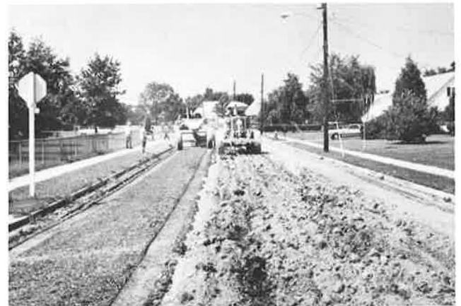
Figure 4. Reconstruction with soil-cement on Virginia street project.
