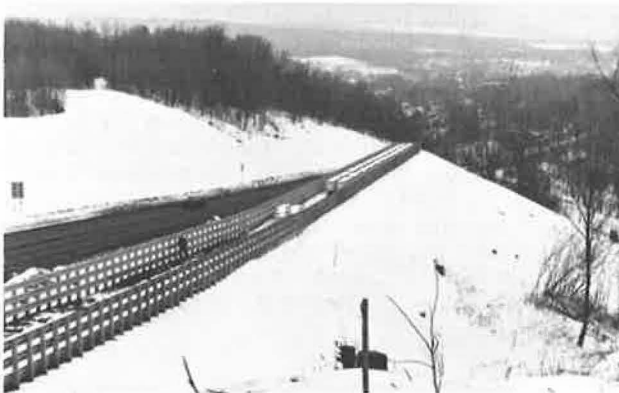
Figure 3. View of arrester system in escape lane showing heavy-post guiderail and sand barrels.
