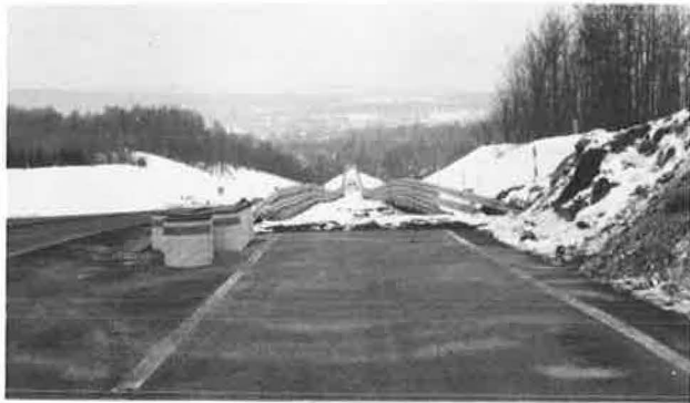
Figure 4. Approach view of arrester system showing impact attenuator to left of entrance.
