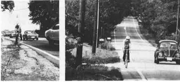
Figure 5. Shoulder before and after smooth-surface treatment.
