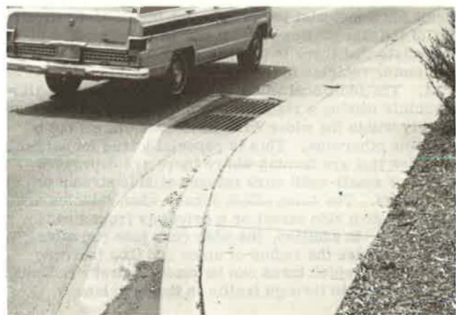
Figure 4. Situation in which a wide curb lane can help bicyclists: avoiding a grate and an overtaking vehicle.
