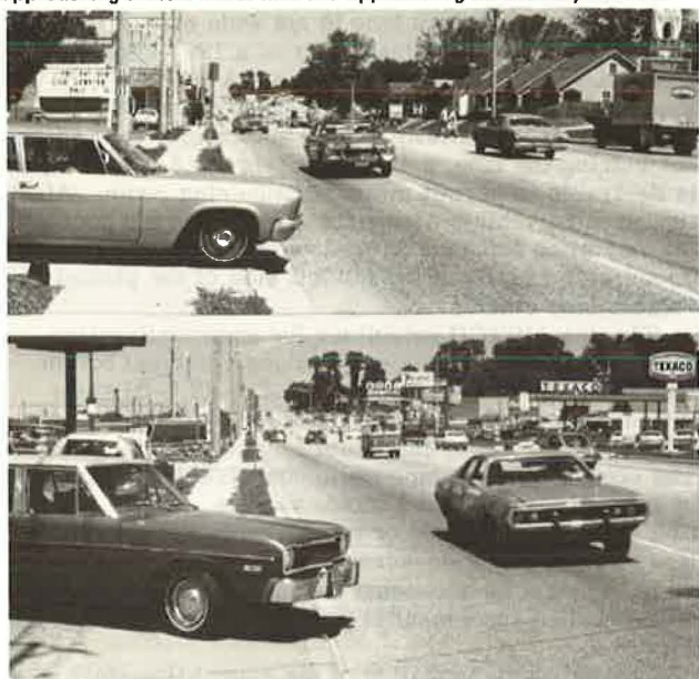
Figure 1. Situation before and after wide-curb-lane treatment: approaching vehicle leaves lane and approaching vehicle stays in lane.
