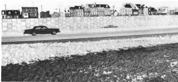
Figure 7. Reinforced-earth wall under construction.
