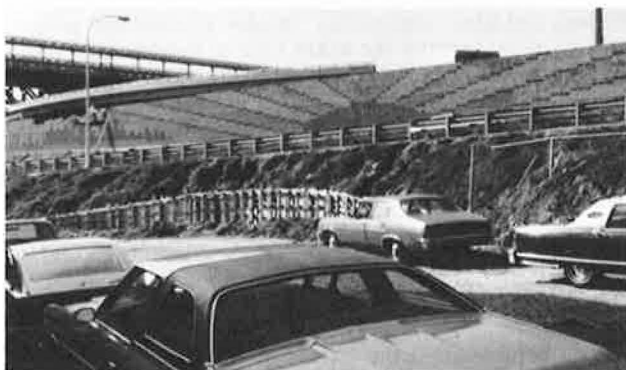
Figure 14. Multicolored concrete-block barrier under construction.
