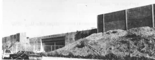
Figure 4. In-place post-and-panel noise barrier.
