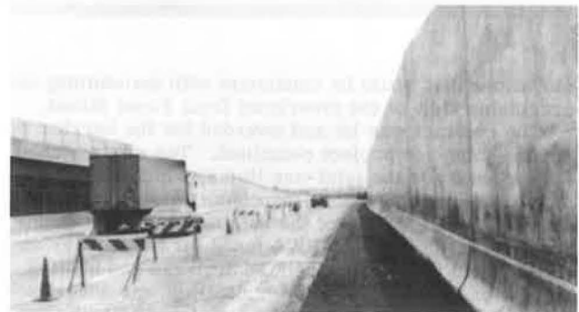
Figure 12. Highway side of brick-faced concrete barrier.
