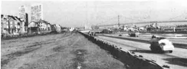
Figure 8. Joint-use area under construction behind reinforced-earth wall.
