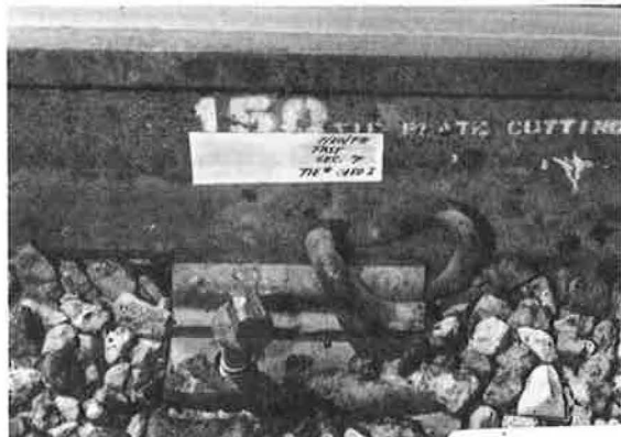
Figure 12. Screw spike out more than 2.5 cm (1 in).
