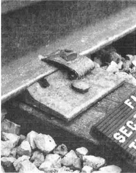
Figure 7. Compression-clip assembly.
