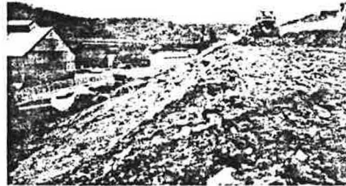
Figure 22. Reconstructed fill in front of root-pile wall.
