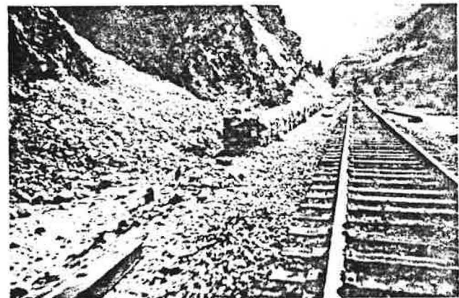
Figure 9. Catchment design using gabion walls.
