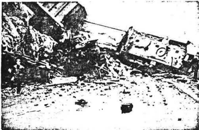
Figure 13. Train derailment caused by train hitting rockfall.
