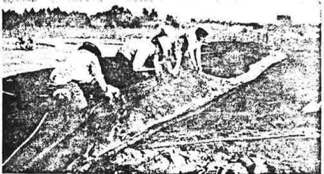
Figure 9. Sewing new fabric strip to existing strip.
