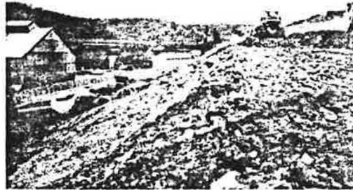
Figure 22. Reconstructed fill in front of root-pile wall.
