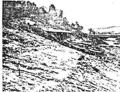
Figure 17. General view before reconstruction.
