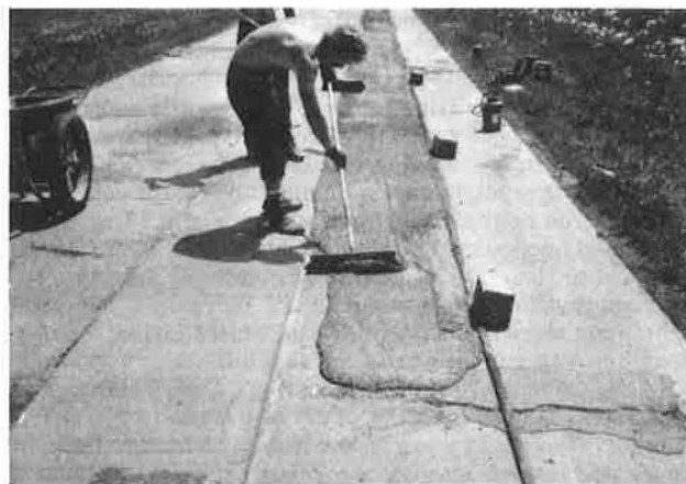
Figure 5. Brooming mortar onto old pavement surface.
