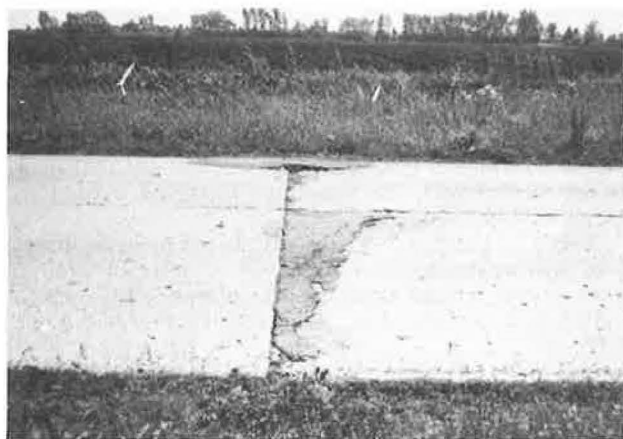
Figure 2. Bituminous patch on existing pavement before overlay.
