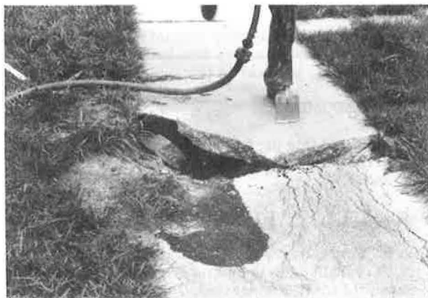
Figure 1. Severe sidewalk undermining.
