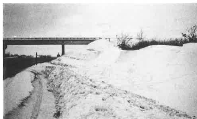
Figure 6. Snowdrifting at grade-separation structure.
