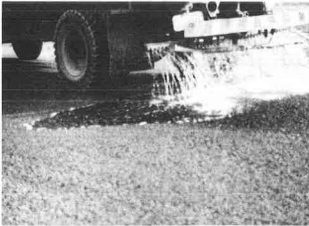
Figure 3. Infiltration test on binder course surface.
