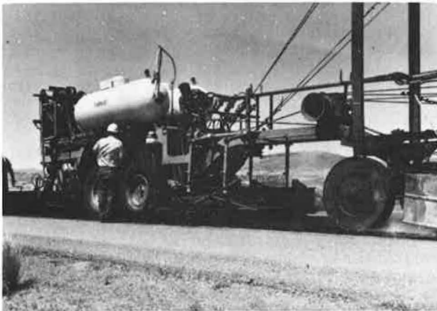
Figure 3. Heater scarification in Arizona.
