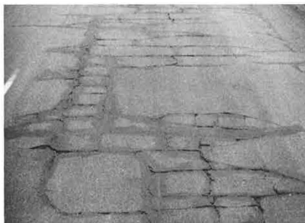
Figure 2. Approximately 35% Cracks
