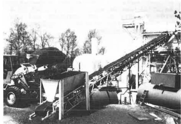
Figure 2. Batch plant modified for mixer heat-transfer method.
