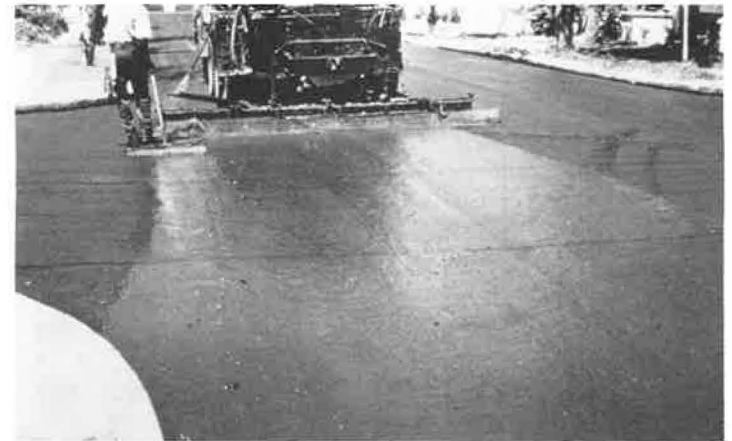
SECOND SLURRY COAT APPLIED OVER PRETREAT- MENT TO FINISH THIS PROJECT
