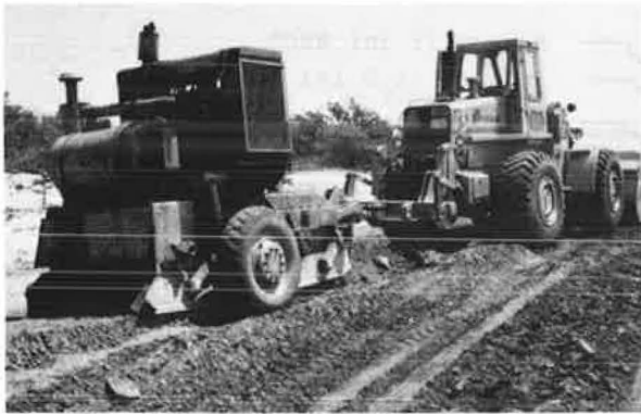
Figure 5. Front end loader towing BROS preparator.
