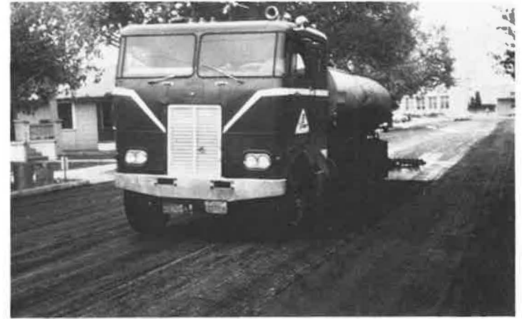
RECYCLING OIL ADDED TO COMPACTED PAVEMENT
