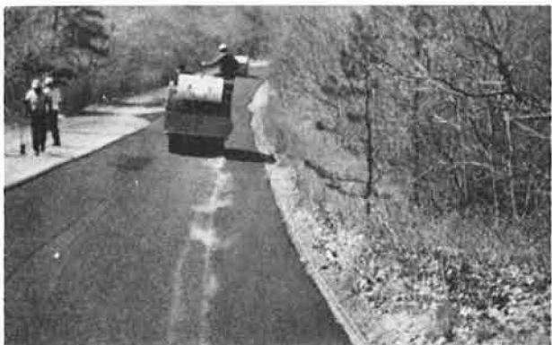
Figure 9. Compacting the wearing course.
