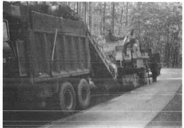
Figure 14. Portable pugmill mixing emulsion with recycle-aggregate blend.
