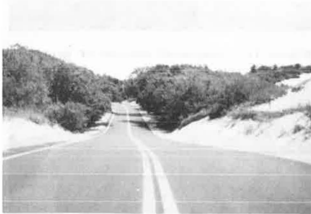
Figure 12. View of completed pavement.
