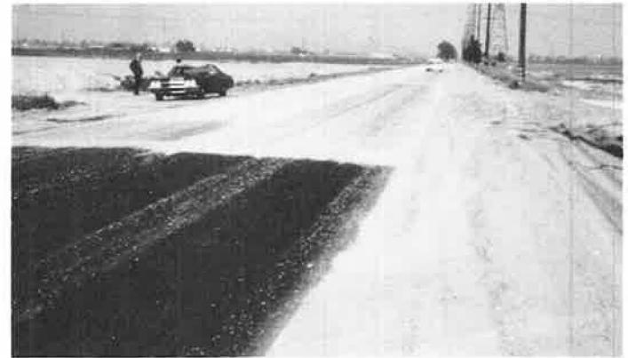
CHIP SEAL WITH UNSEALED CONTROL SECTION IN FOREGROUND
