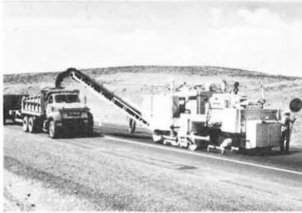
Figure 1. Cold milling machine.
