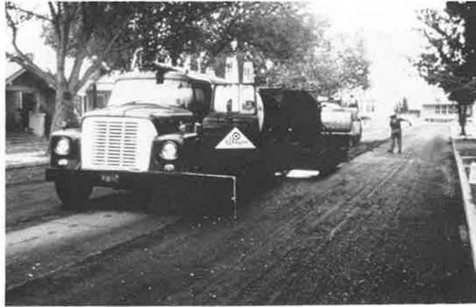
HEATER SCARIFYER, RAKERS AND ROLLER FORM CITY MAINTENANCE PROGRAM
