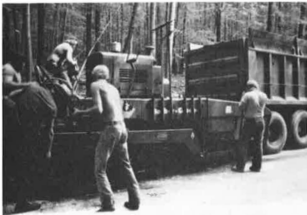
Figure 15. Placement of recycled material.
