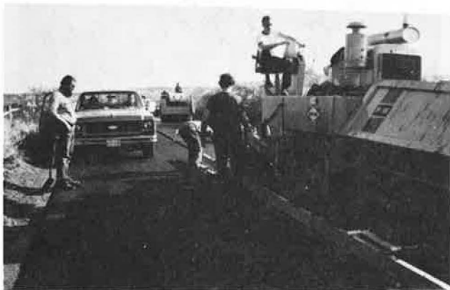
Figure 9. Compacting the wearing course.
