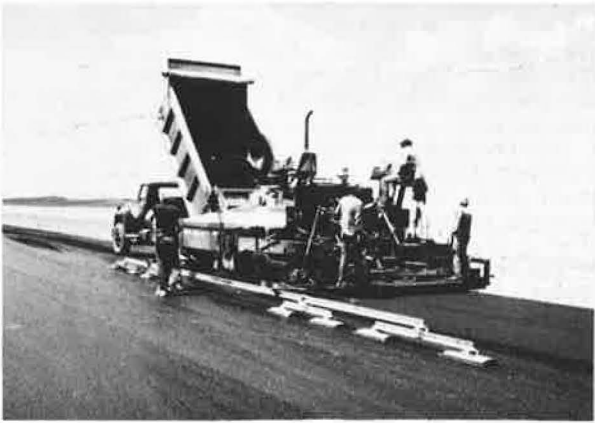
Figure 6. Laying mix containing reclaimed asphaltic material.
