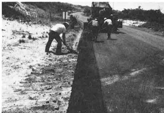
Figure 11. Completed section of berm.
