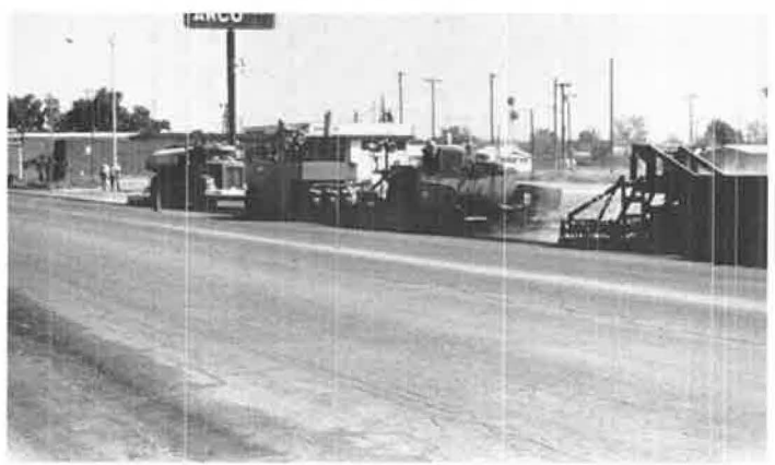
SCREED, RUBBER TIRED COMPACTOR AND OIL SPREADING TRUCK
