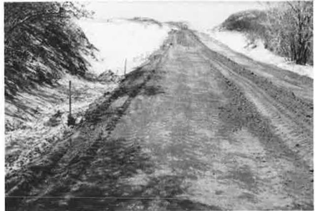
Figure 7. Partially compacted recycle material.
