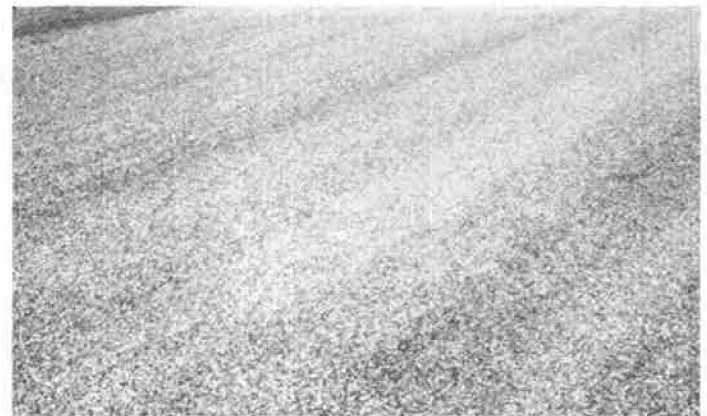
CLOSEUP OF 3/8" MAXIMUM CHIP TREATMENT ON RECYCLED PAVEMENT
