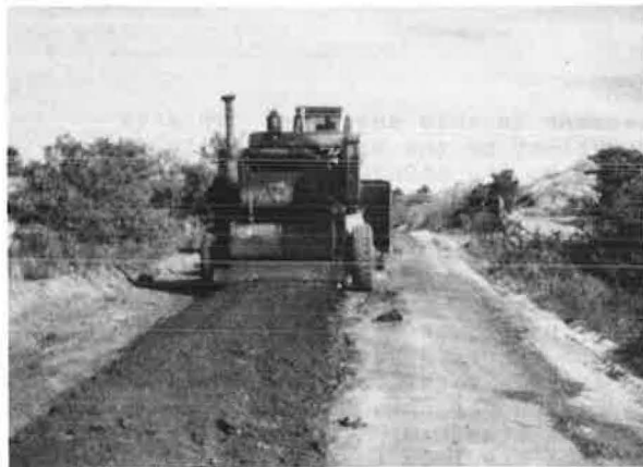
Figure 6. BROS preparator pulverizing windrowed material.
