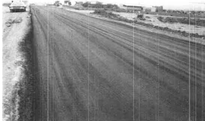
COMPACTED SURFACE AFTER RECLAMITE APPLICATION
