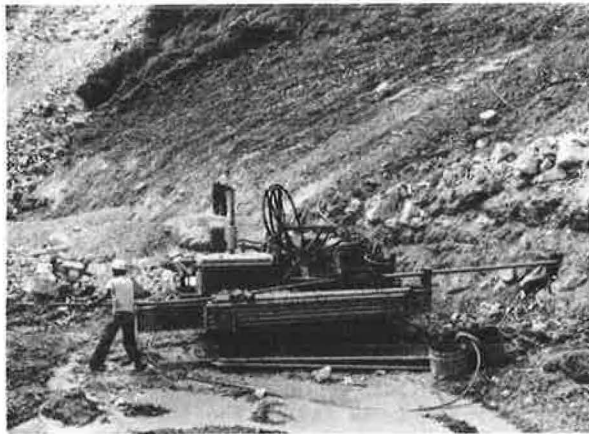
Figure 4. Horizontal drilling rig.
