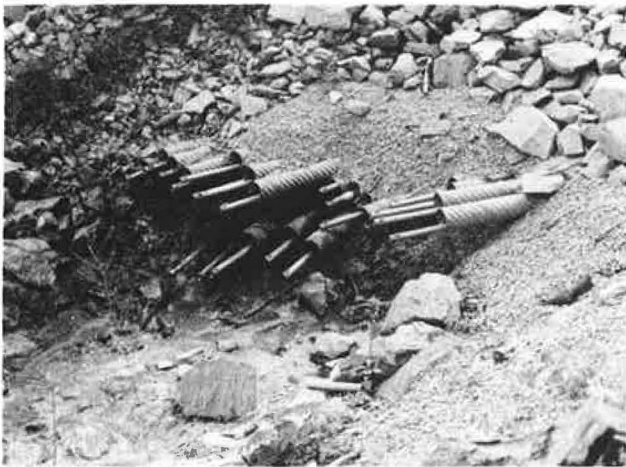
Figure 6. Completed horizontal drain installation at pad B.
