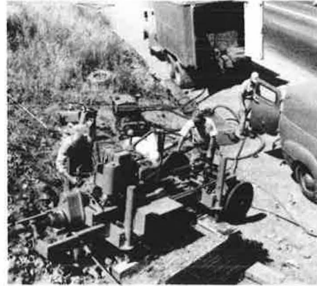
Figure 4. California horizontal drill rig, June 1954.
