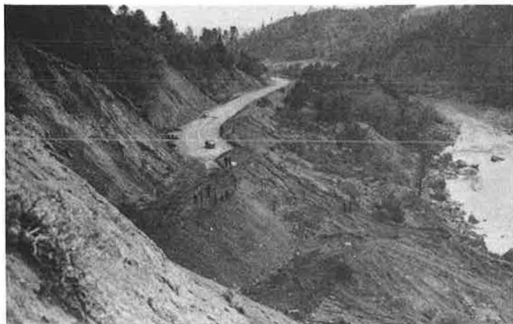
Figure 7. Cloverdale landslide and slipout, December 1941.
