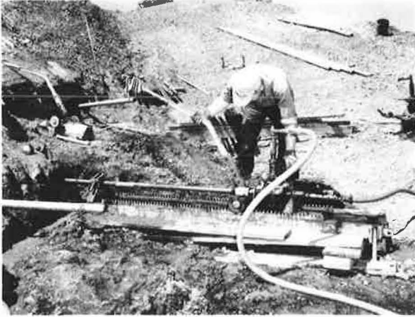
Figure 1. Hydrauger, first used in 1939 to install horizontal drains by CDH.
