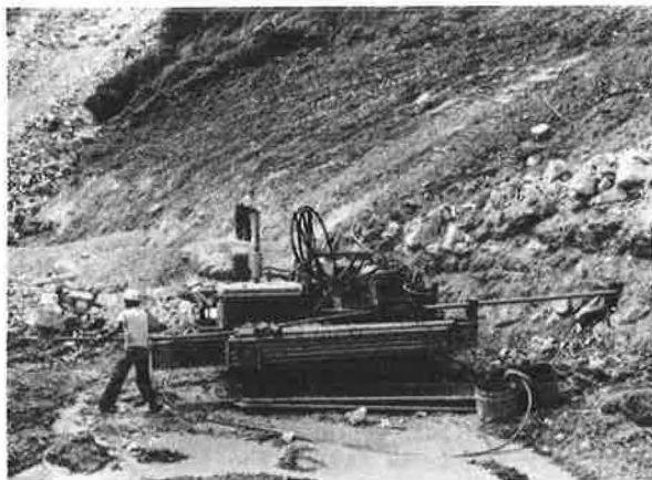
Figure 4. Horizontal drilling rig.
