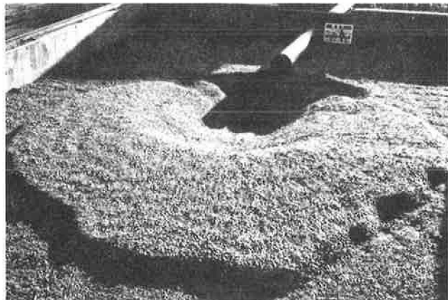
Figure 3. Scour hole in uniform gravel material.
