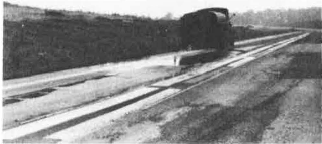
Figure 5. Preparation of test site.
