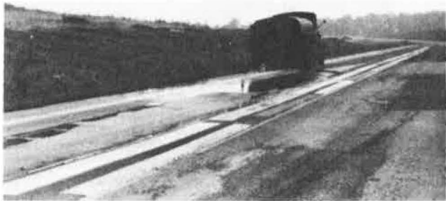
Figure 5. Preparation of test site.
