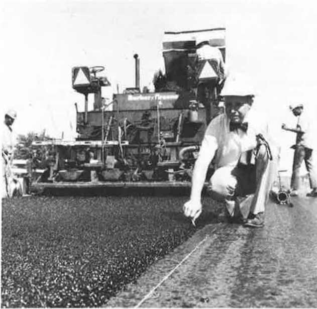
Figure 1. Open-graded asphalt friction course.
