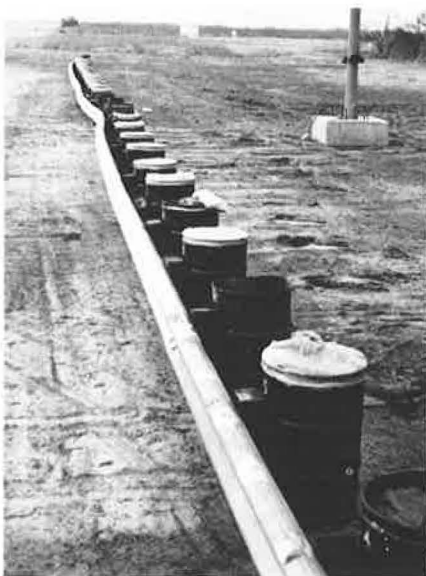
Figure 15. SBW3 installation restored after test 3825-3.
