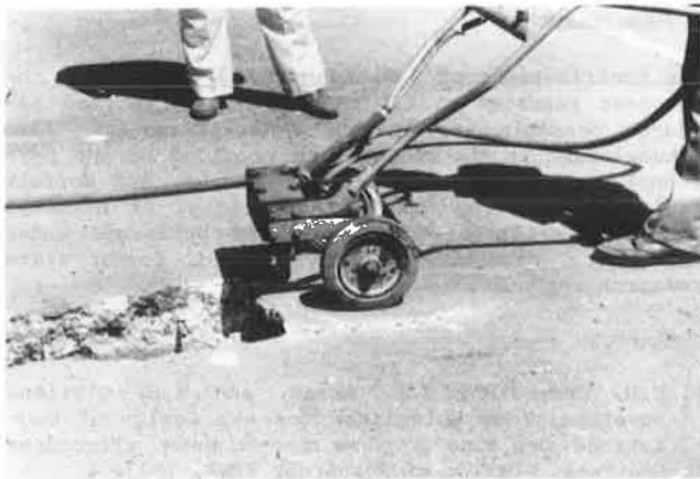
Figure 2. Crack chaser in operation.
