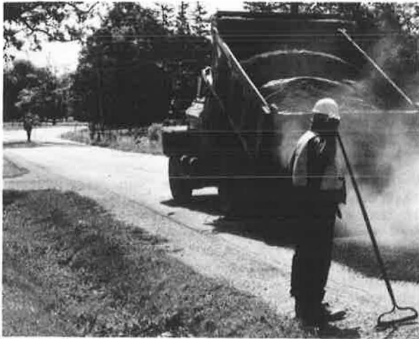
Procedures for Placing and Spreading Hot or Cold Mix Asphalt (Machine Patching)
