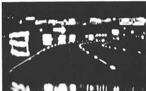
Figure 3. Visibility of raised pavement markers.
