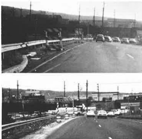
Figure 2. Type 3 barricades: (top) fourth barricade blocked from view and (bottom) fourth barricade visible over top of car.
