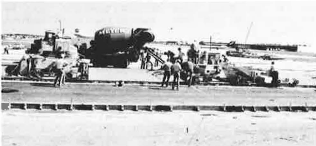
Figure 3. Paving train in operation.
