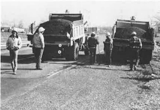
Figure 2. Trucks carrying different mixtures for comparative field evaluations.
