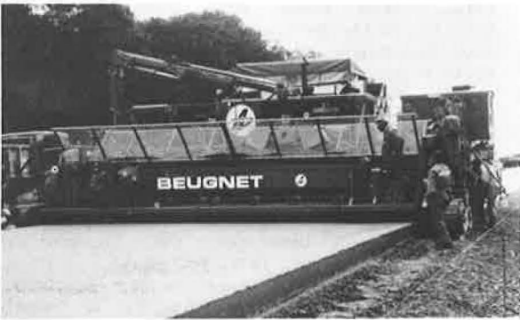
Figure 5. Séléstat bypass under construction in 8-m-wide sections.
