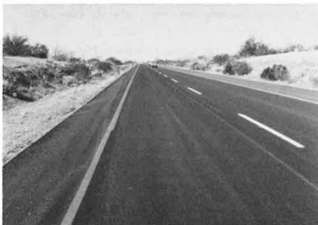
Figure 2. Ability of ACFC to hide cracks in known cracking area.
