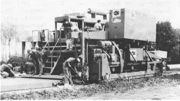
Figure 4. Slip-form paver at work at Bernissart site over 3.5-m width.
